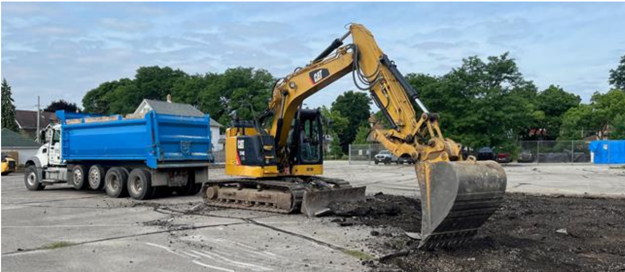
Removing Asphalt
