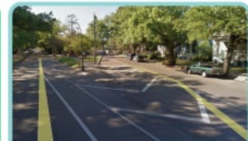
d Bayou Road Curb Extension
