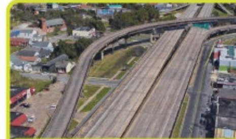
a North Claiborne Avenue Detention Basin
