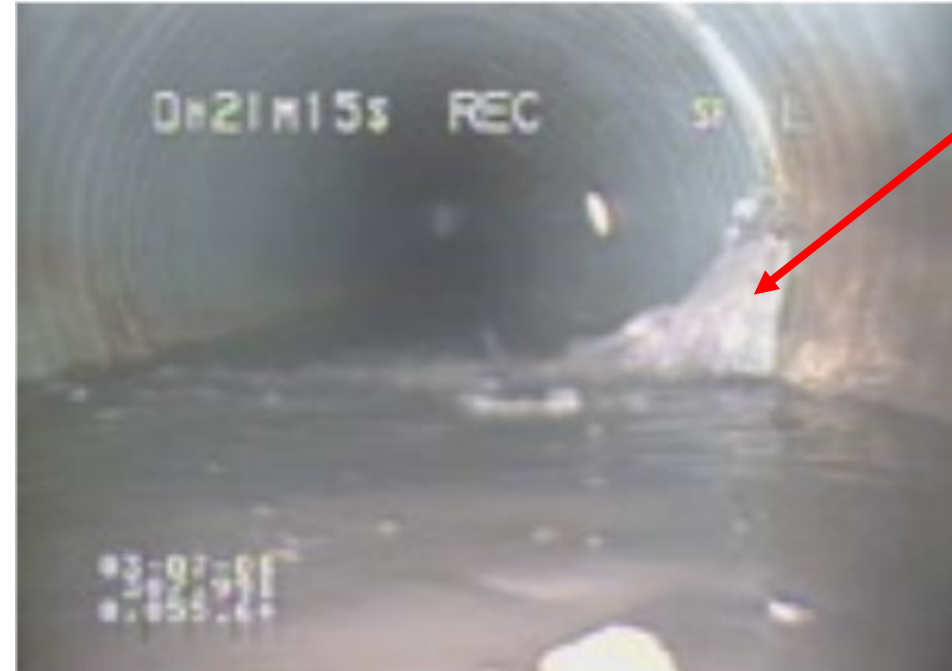
Infiltration through pipe joint
