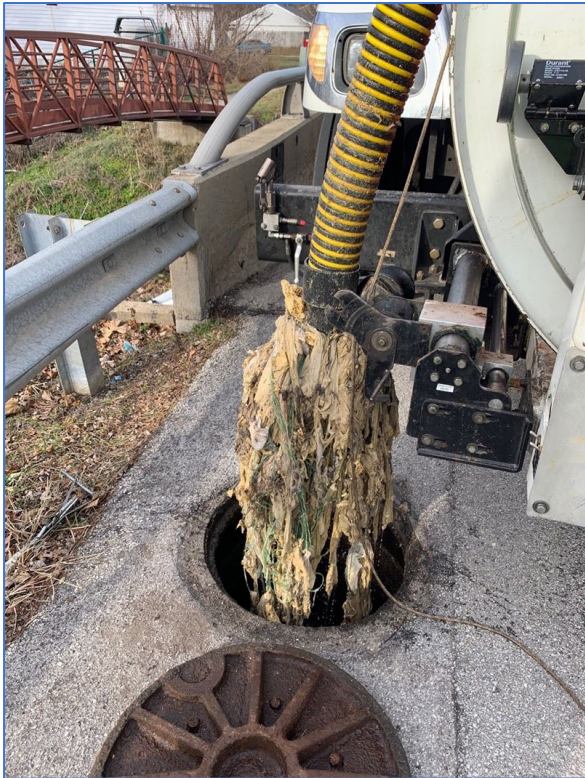
Vac removing clog of rags and grease
