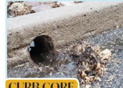
Circular core drilled through curbing that serves as an inlet or outlet
