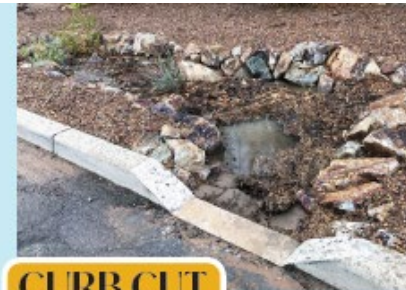
Removed section of curbing that serves as an inlet or outlet
