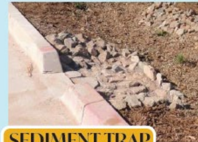
Rough area at inlet that allows sediment to settle before water enters a basin
