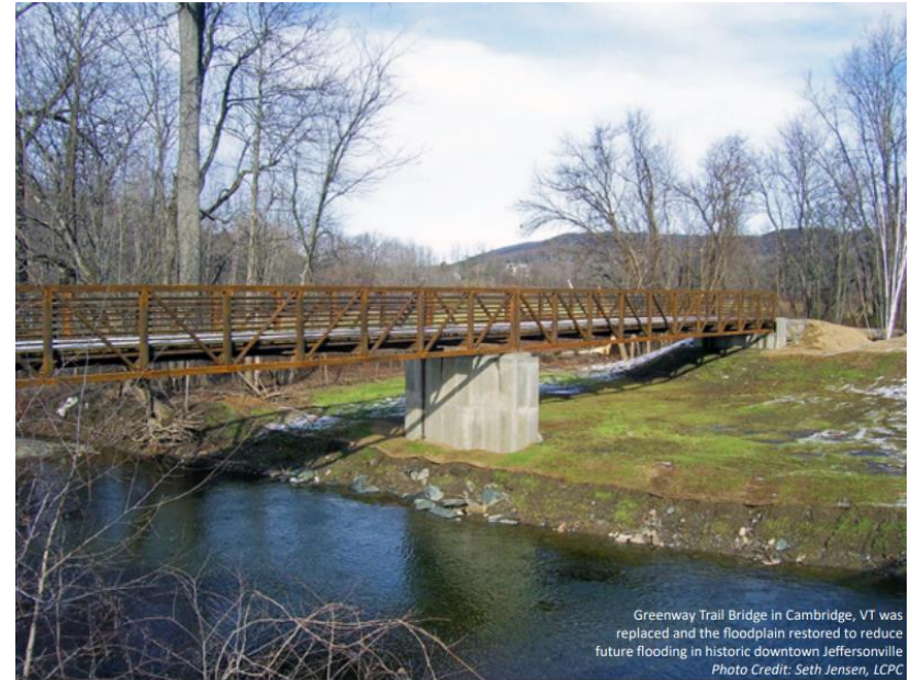
Greenway Trail Bridge in Cambridge, VT
