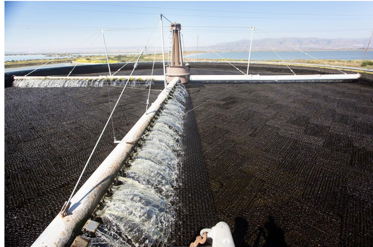
Photo of a Trickling Filter.
