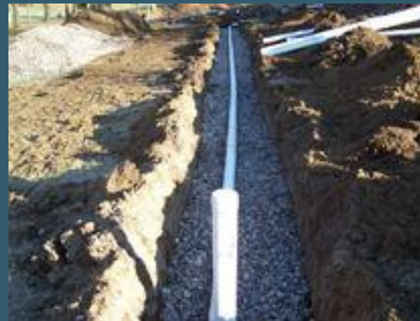
Installing lateral in gravel filled trench
