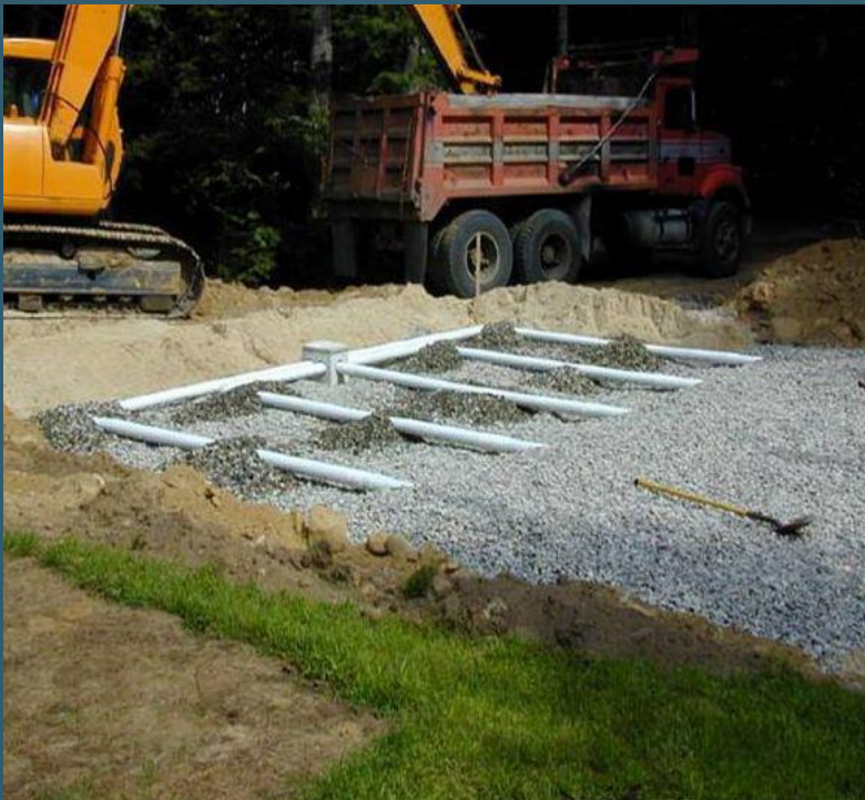
Installing distribution laterals
