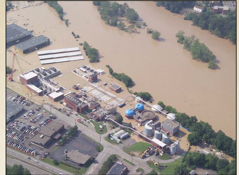
City of Binghamton/Village of Johnson City Joint Sewage Treatment Plant 2006
