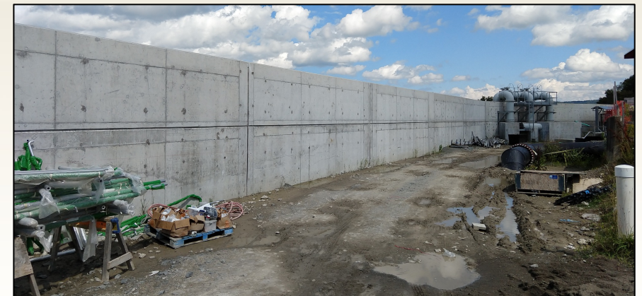
New Flood Wall along Susquehanna River
