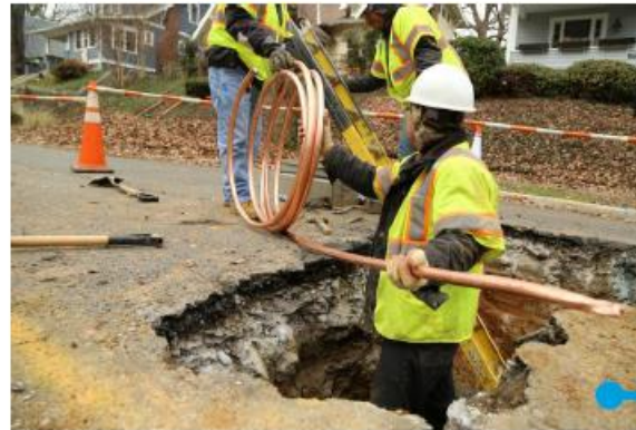
Lead Service Line Inventory and Replacement
