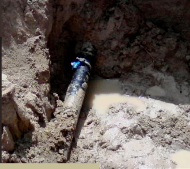
LEAKAGE ON MAINS
