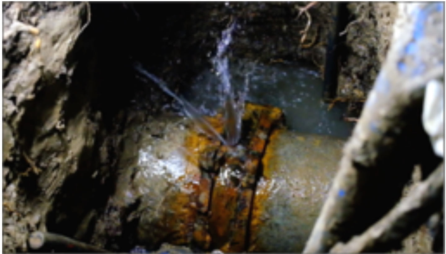
Asbestos cement water main leak.
