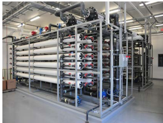
Nano Filtration Membrane System (Pilot Butte, Saskatchewan, Canada)
