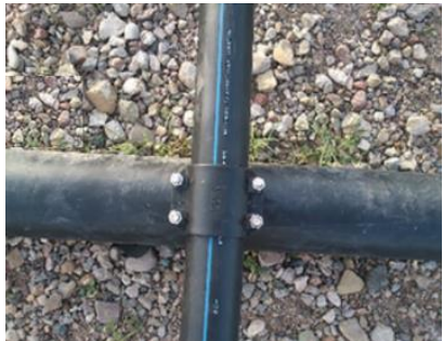
A short section of pipe to keep the diffuser laterals from twisting
